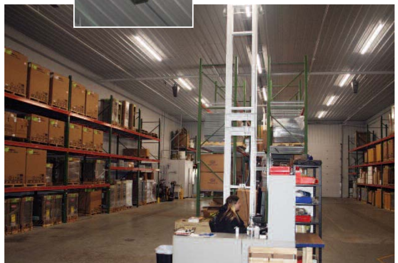
D-STRAT™ fans in the 20-foot high ceiling of 5,500 square-foot warehouse direct heated air down to occupant working zones.
