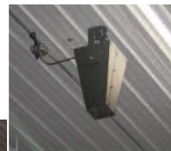
D-STRAT™ fans in the 20-foot high ceiling of 5,500 square-foot warehouse direct heated air down to occupant working zones.
